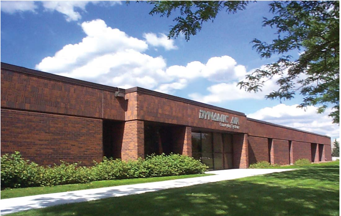
Dynamic Air Inc. Sede Central, St. Paul, Minnesota, USA
