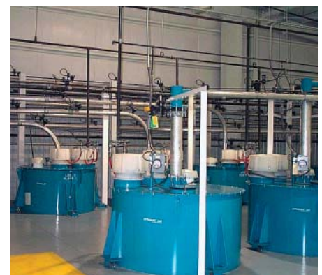
Multiple 20 cu. ft. (0.6 cu. m) surge bins with Modu-Kleen® 669 bin vent filters.
